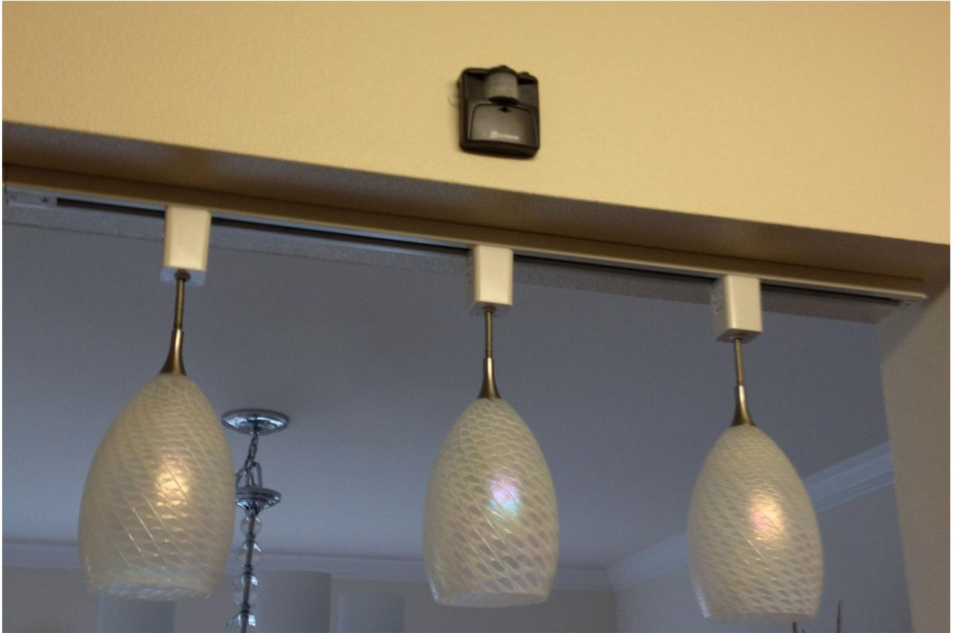
**Figure 1.** Motion sensor installed in the home of a study participant. This figure illustrates how a motion sensor used in the study looks after it has been installed in the kitchen of a residence.
